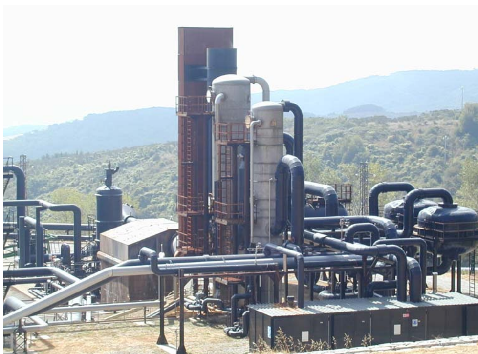
Figure 12.1 The ENEL proprietary AMIS hydrogen sulphide and mercury emission abatement system installed at the 20 MW e Bagnore 3 geothermal power station, Tuscany, Italy. (Photo by Aldo Baldacci, ENEL).
