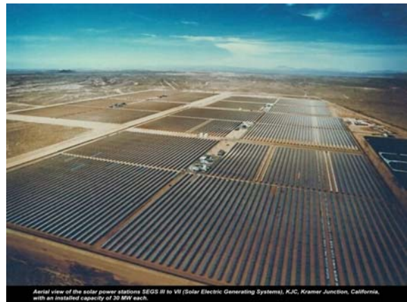
Aerial view of the solar power stations SEGS III to VII (Solar Electric Generating Systems), KJC, Kramer Junction, California, with an installed capacity of 30 MW each.
